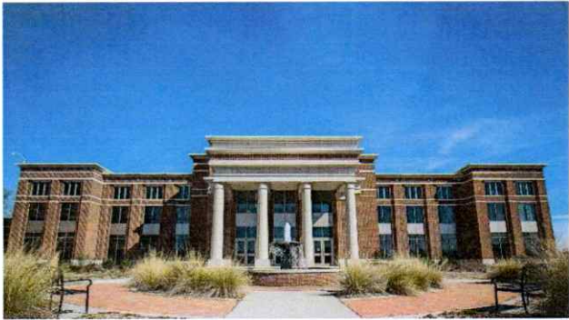
3. West Elevation: Courts Building
