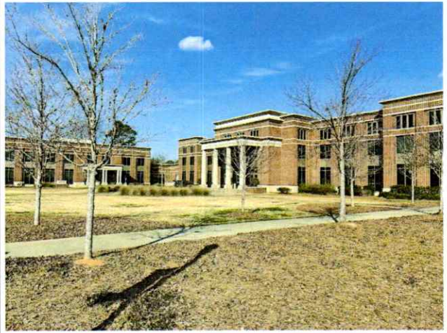
2. Overview of Facility. Two 2-story buildings and a connected 1-story breezeway.
