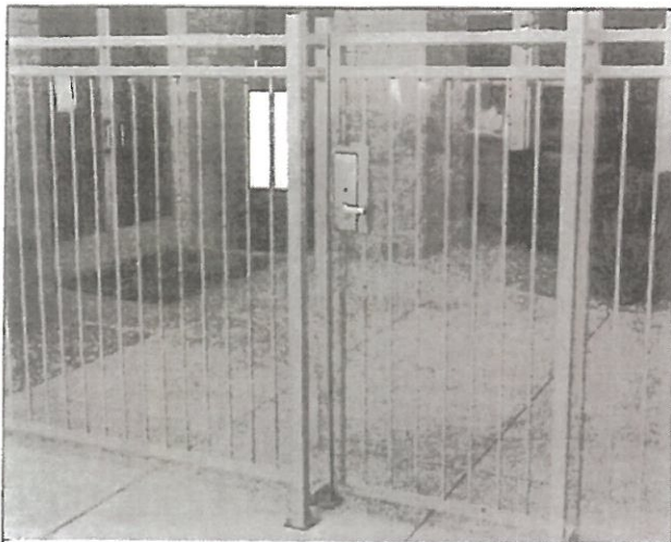
Commentary Figure 305.2.6(2) VIOLATION—BARRIER (FENCE) HORIZONTAL MEMBERS TOO CLOSE
