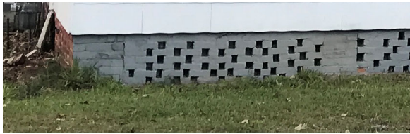
Brick piers infilled with brick in a lattice pattern
